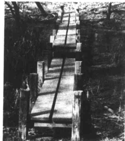
OMAHA — Footbridge donated by Club 124.
